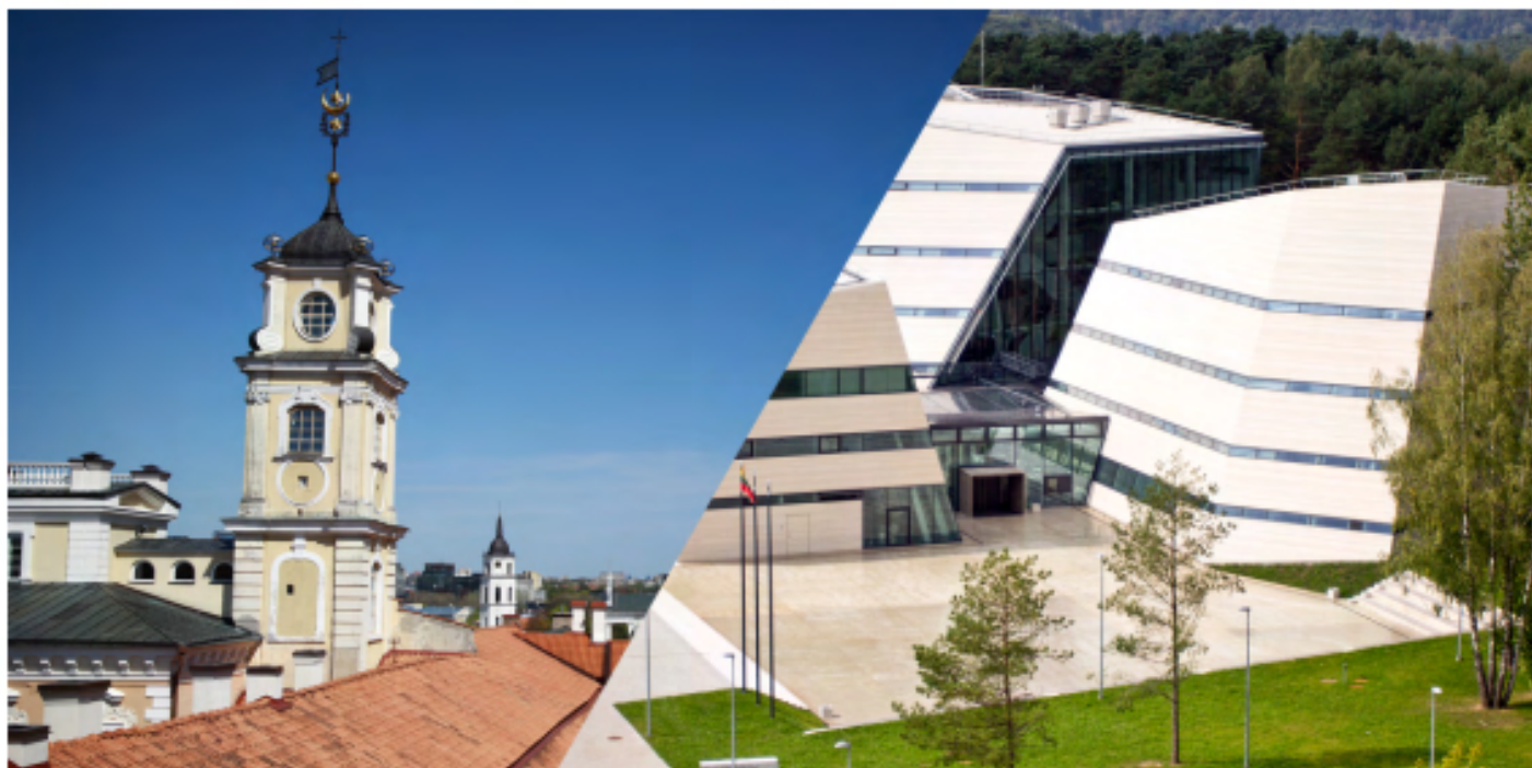
The buildings of Vilnius University Library in Vilnius Old Town and Sauletekis
